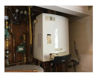
Corrosion was observed on the water distirbution pipes for the hydronic heating system. No water leaks were observed at the time of the inspection.
