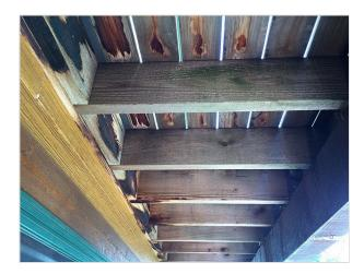
A few of the joist hangars on the middle deck appear to be coming loose. Recommend repairs by a qualified contractor.
