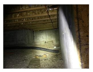
The sub-floor above the crawlspace lacks insulation. Adding insulation may help regulate the temperature of the living space above the crawlspace and may assist in preventing moisture intrusion.
