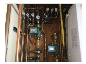
Corrosion was observed on the water pipes for the water heater. No water leaks were observed at the time of the inspection.
