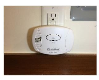
Per Colorado state law, carbon monoxide detectors are required to be installed within 15 feet of all sleeping areas. No carbon monoxide detectors were observed installed within 15 feet of the sleeping areas on the upper level.
