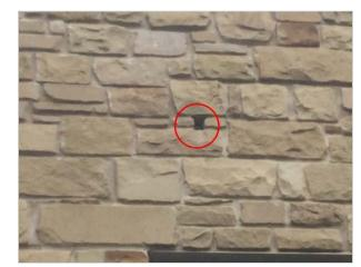
Assumed secondary condensate drain line did not penetrate to exterior
