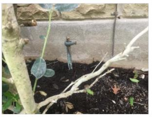
Grounding electrode not fully driven
