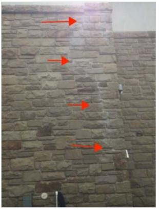
Prior mortar crack repairs
