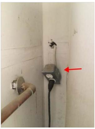
Receptacle not attached to wall
