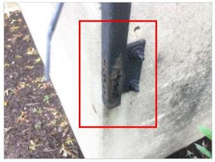
Rust at back porch steel railing spindle
