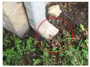
Clogged downspout with missing splash block
