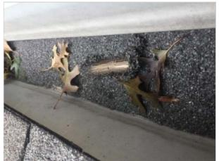
1/8-inch granule accumulation and debris in gutters
