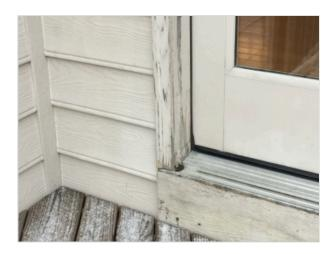
Loose siding was present on the left side of the home. The siding should be reattached.
