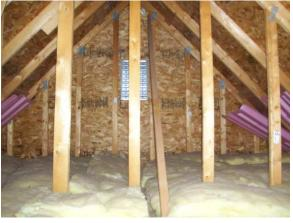
Because of the configuration of the framing and absence of a catwalk, which limited access, it was not possible to inspect all areas of the attic. There was no moisture visible in the attic space. The absence of visible indications of moisture is not necessarily conclusive evidence that the roof is free from leaks. The only way to be sure a roof does not leak is to inspect the underside of the roof during a heavy rain. There were no major visual defects observed in the attic or roof structure.
