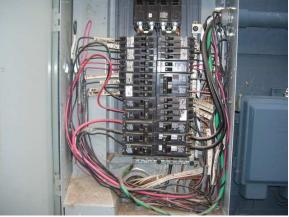
The branch circuits within both panels were copper. These branch circuits and the circuit breakers to which they were attached appeared to be appropriately matched. The visible house wiring consisted primarily of the Romex type and appeared to be in good condition.
