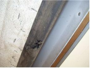
• Air gaps were observed at the rear exterior "man" door and the weather strip was damaged at this door.
