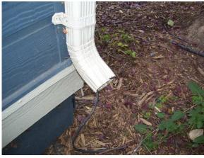
• Some of the heat tape at the back of the home was not installed in the gutter.
