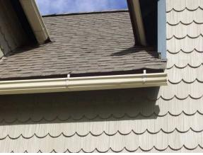
There was light curling and moderate surface wear observed on the roof shingles at the time of the inspection. These conditions indicate the roof shingles were in the middle stages of their useful life. This visual roof inspection is not intended as a warranty or an estimate on the remaining life of the roof. Any roof metal should be kept well painted with a paint specially formulated for the use. There were no major visual defects detected on the exterior of the roof.
