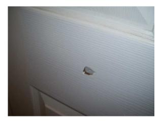
There were no door stops or the door stops were damaged at many of the doors. Door stops should be installed and/or repaired to help prevent possible blemishing of the walls that could be caused by door handles.
