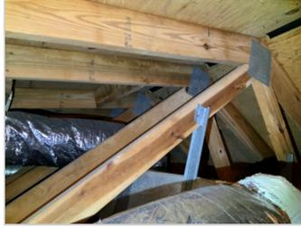
**Cut truss(es) observed in the attic.** This is a support/installation/damage concern. Typically, truss modifications/repairs are to be approved by the manufacturer or structural engineer. Modifications to trusses can alter the design load. Recommend review and repairs as directed by a structural engineer with repairs performed by a qualified contractor.
