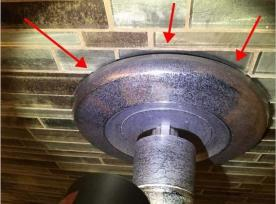
The master shower control plate should be sealed at the wall.
