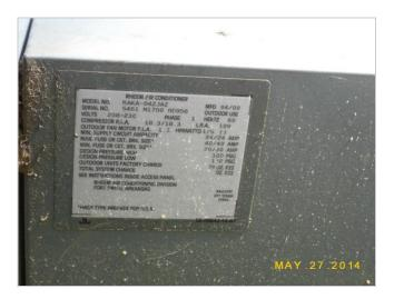
The electric outdoor air conditioner condensing unit for the second level was a Rheem, model # RAKA-060JAZ and serial #5721 M1800 13203. The unit was located at the left side of the home. This unit is approximately 14 years old. The cooling system was found to be functional.
