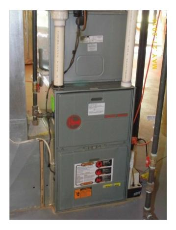
The second level of the home was heated by a Rheem propane gas forced air furnace, which is 14 years old. The unit was located in the attic of the home. The heating system was found to be functional.
