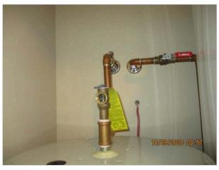
Due to the age of the water heater (17 years) it is considered to be past the end of its life expectancy and therefore failure is possible without warning. The water heater may need to be replaced in the near future.
