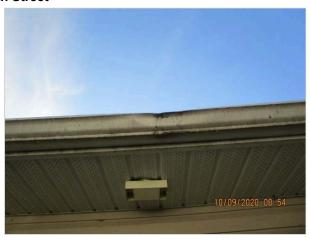
There were eavestroughs and downspouts on the home that were in need of cleaning to the extent that they were ineffective in their current condition. It is recommended that the eavestroughs be cleaned to prevent them from overflowing.
