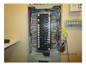
The electrical service appeared to be adequate for a typical single family needs. Alarms, electronic keypads, remote control devices, landscape lighting, telephone and television, and all electric company equipment are beyond the scope of this inspection. There were no major visual defects observed in the visual electrical system.
