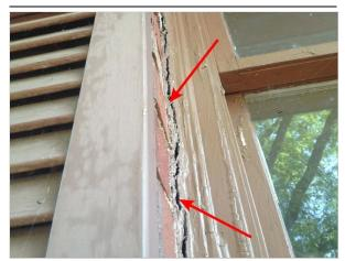
Wood rot and/or decay damage found on the roof fascia/soffit boards in the following locations of the property:
