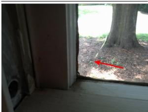
• A representative number of the windows were painted shut and could not be operated to verify operation or check for defects. The window(s) need maintenance to free them for opening and further inspection.
