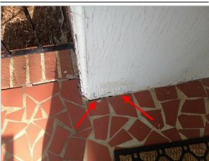
• The paint was peeling of exterior surface at the multiple locations-conducive for wood deterioration. Needs proper repair by a painting contractor.
