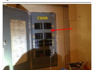
• The panel ground to a water pipe has been nullified by a plastic water main. Either an auxiliary ground should be established, or the panel should be regrounded. Needs repair by a licensed electrical contractor.
