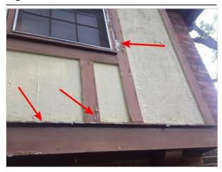
Caulk is missing and/or deteriorated between the window jambs and brick walls - seen around front left window.
