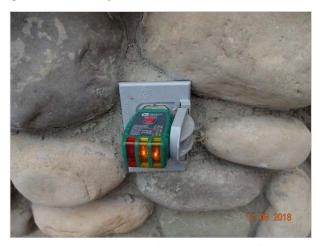
The GFCI outlet located on the exterior, to the right of the garage is defective and should be replaced by a qualified electrician.
