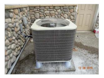
The heat pump unit appeared to be have leaked prior to the time of inspecition. Due to the cold temperature, the water has frozen over and the unit was surrounded by ice. If the unit continues to function in this state, severe damage to the unit could occur. It is highly recommend that a licensed HVAC contractor be contacted for further evaluation and repair recommendations before further use.
