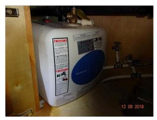
There was no drip leg installed on the T&P valve of water heater #2. The drip leg directs water from the T&P valve toward the floor. A drip leg terminating within six-inches of the floor should be installed.
