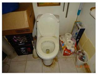
Water marks with minor surface damage was noted on the main level bathroom floor. The water marks
