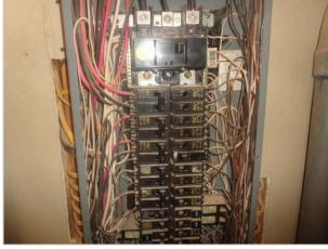
The visible house wiring consisted primarily of the Romex type and appeared to be in good condition. An electric service grounding system was installed. Service grounding requirements have changed many times over the years. The grounding system for a 30-year-old electric service is different from that of a 10-year-old service. The inspection does
