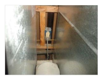
One or more exterior outlets were not properly covered. Outlet covers designed for use in wet locations should be installed on all exterior outlets.
