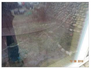
One or more of the insulated window panes throughout the home had a defective thermal seal. A defective
