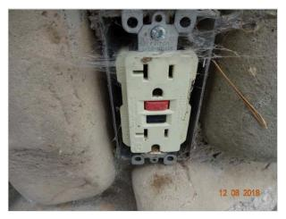
One or more missing switch or outlet covers were noted in the basement. All switch and outlet boxes should be properly covered to avoid a shock hazard. Electrical related repairs should be performed by a qualified electrician.
