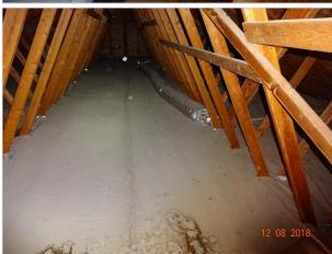
• Water marked or damaged roof decking was noted in the attic. The marks appear to be the result of previous leaks. Repairs to the affected areas are not required. No immediate action is necessary. It is recommended that the attic be monitored for further leaks and be repaired as needed.
