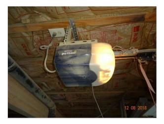
The Overhead Door brand electric garage door opener was not able to be tested. The automatic safety reverse on the garage door was not tested because the garage door opener was not functional at the time of inspection. The functionality of remote transmitters, keyless entry or other opening devices is not tested during the home inspection.
