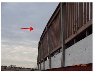
• There were minor damaged and cracked boards noted around the right and rear sides deck. Repairs should be made as desired.
