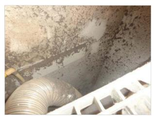
· There was no visible dryer vent installed. Clothes dryers should be vented to the exterior of the home. Consult
