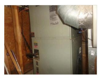
Examination of heating systems is mechanically limited since the unit cannot be dismantled to examine all of the interior components. The electric heating elements can and will fail. Heating elements fail just like light bulbs; they are working one minute and not the next. The symptom of a failed heating element is usually lukewarm heat. The inspection does not include a heat-loss analysis, heating design or adequacy evaluation, energy efficiency assessment, installation compliance check.
