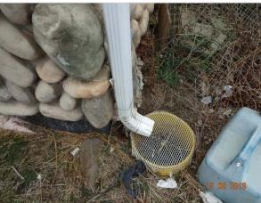
• All of the downspout (s) were draining at or too close to the base of the foundation. All roof drainage should be directed at least six feet from the base of the foundation.
