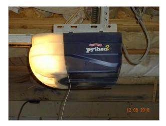
The Overhead Door brand electric garage door opener was tested and found to be functional. The automatic safety reverse on the garage door was tested and found to be functional. The functionality of remote transmitters, keyless entry or other opening devices is not tested during the home inspection.
