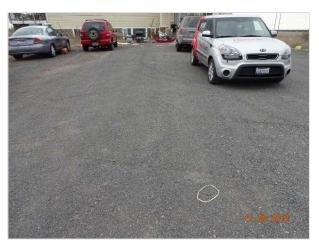
• There were uneven areas and potholes noted on the front and rear sides of the gravel driveway. These conditions can be a trip hazard and could potentially cause damage to a vehicle. It is recommended that these areas be repaired using a suitable or similar surfacing material to "feather" the out-of-level conditions to make a smooth transition. Contact a qualified contractor for further recommendations and repairs.
