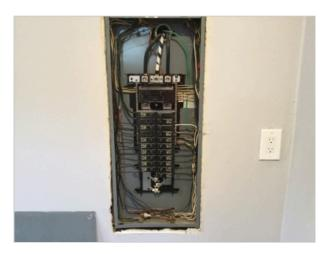
An open knockout was observed in the electric service panel, creating the potential for electric shock. All service panel openings should be covered to prevent access to high voltage and risk of electrical shock. Electrical related repairs should be performed by a qualified electrician.
