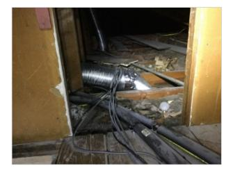
Electrical junction box not properly fastened.
