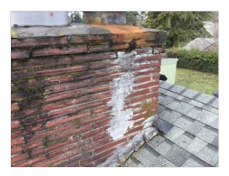
**The chimney is missing a rain cap**. A rain cap should be installed to prevent excessive water intrusion and deterioration of the chimney and its components.
