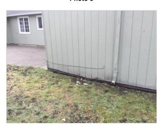
A loose gutter mount was observed at the time of the inspection. This is a common condition and is caused by expansion and contraction, along with the freeze thaw cycles that we experience in this area. The mounts should be resecured and the underlying fascia checked for damage.
