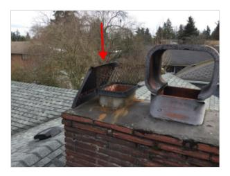
**The flashing around the chimney requires repair.** Flashing is a critical component that helps prevent water intrusion. At the time of repair, the technician should investigate the area for any previous water intrusion or damage.
