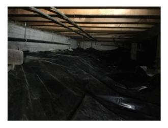
A section of floor structure is damaged from previous water intrusion. It was not clear whether the water intrusion has ceased. Monitor the area for any additional water intrusion, and repair as needed.
