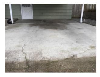
**Areas of the driveway have settled.** This condition indicates a possible void under the driveway. Driveway settling has led to potential tripping hazards. The areas should be monitored and repaired as needed.
