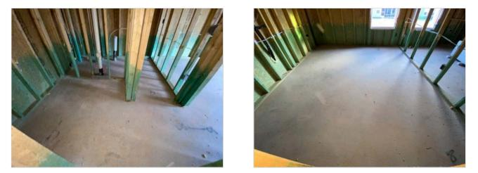
Around the foundation, the foam insulation panels are damaged. The purpose of the insulation is to knock down heat gain or loss from the home through this concrete and help keep the floor temperature more stable. Hve the builder repair the panels as needed.
