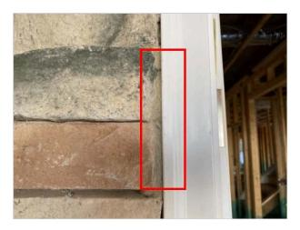
At the stone veneer around the home, there is at least one area where the mortar is incomplete. This can allow moisture and pest intrusion. Have the builder repair everywhere needed.
