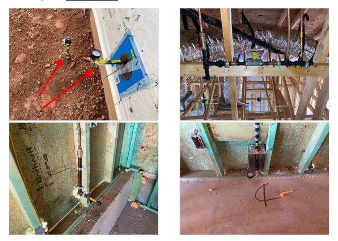
At the incoming gas line, the test gauge is reading 0 psi. This may mean the static pressure test has failed, indicating a leak in the system. Also, the gauge at the kitchen gas pipe reads 5 psi. Both gauges cannot be correct, but either reading indicates a possible test failure. Prior to insulation and drywall work, have the builder ensure the gas piping is properly installed and passes the static pressure test.
