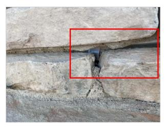
At the front of the home, there is one area where the house wrap is torn. Have the builder repair and tape the wrap as needed prior to siding installation.
