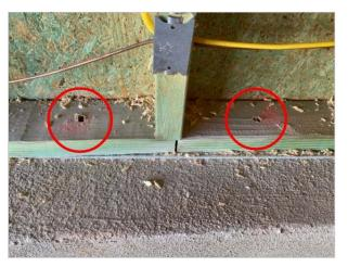
At the family room/garage perimeter wall, there is a gap where daylight is visible. Have the builder seal all gaps and holes in the perimeter walls prior to interior finish work.
