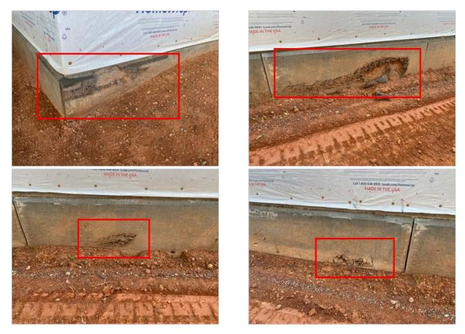
At several places, the concrete slab is damaged. Have the builder repair the slab as needed prior to interior finish work
