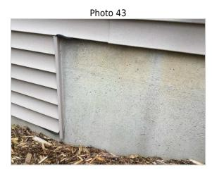
Small cracks were observed on the foundation. The cracks were 1/16th-inch or less in width. The homeowner should monitor these cracks for any changes, and if changes are noted, should contact a structural repair company for further analysis. Below-grade cracks are highly susceptible to water intrusion during times of heavy rain. Water staining from previous water intrusion was not visible. HomeTeam recommends sealing these cracks if a watertight basement is desired.
