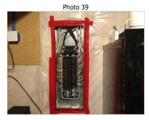
**Corrosion was observed on components in the electric panel**. Corrosion on terminal screws and wires can result in overheating of terminals and possible arcing problems in the panel. HomeTeam recommends that a licensed electrician repair and further evaluate the condition of the electrical panel.
