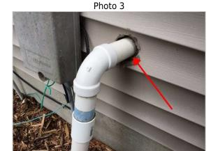
Suggest caulking around pipe on left side of structure to prevent insect/water intrusion.
