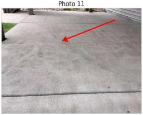
Recommend sealing crack in patio to prevent water intrusion.
