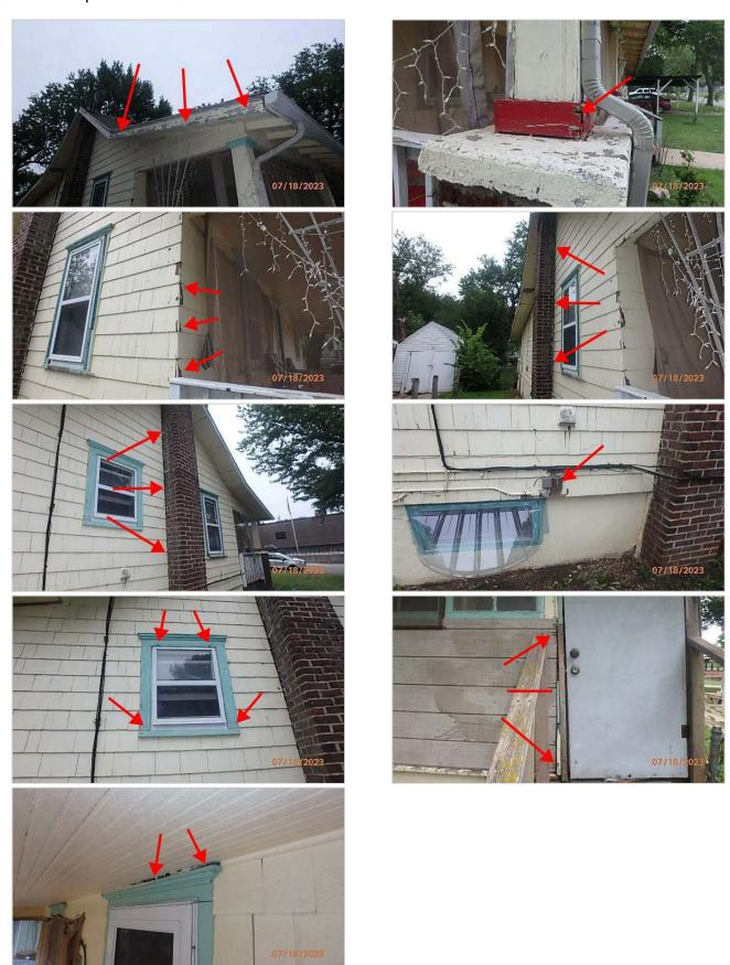
There was some decay observed on the exterior wooden elements in a few places. These are in need of some repair.
