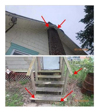
It is unlikely that every incident of decay or dry rot on the exterior of the home were seen by the inspector. The visible evidence of decay may be difficult to spot when covered by paint, hidden from view by vegetation, or on areas of the home not immediately visible to the inspector.
