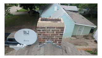
The chimney is in need of service to seal up the flashing around the base, repair the crown, and install a rain cap.
