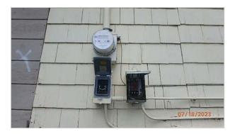
The electrical service wires located just outside the weather head have damage to the insulating jacket caused by age. These wires are in need of replacement from the overhead connection to the meter to eliminate potential short circuiting or accidental contact.
