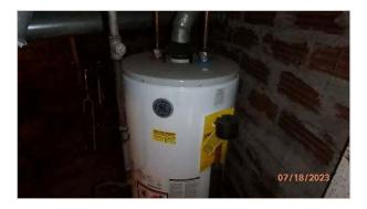
Average service life for water heaters is generally considered to be 10-12 yrs, although there are varying grades of heaters. It is not uncommon to see water heaters that are 20 or more years old that are still functional.
