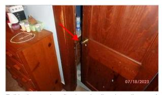
Full bathroom door (latch and strike plate alignment)
