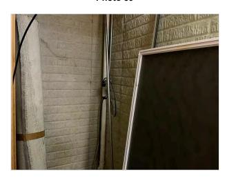
The sump pump appears to be missing a check valve. Check valves prevent the backflow of water back down into the sump crock which can overwork the sump pump and cause early failure. HomeTeam recommends consulting with a qualified plumber to instal a check valve in the discharge pipe.
