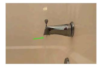
The shower head for the upstairs hallway bathroom is loose where it attaches to the wall. The pipe should be secured and the area sealed in order to prevent water intrusion.
