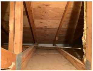
No insulation observed in garage ceiling or rafters
