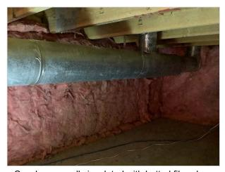
Crawlspace walls insulated with batted fiberglass
