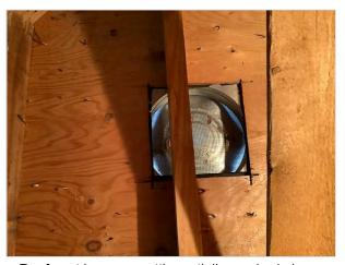
Roof vent in garage attic partially crushed above
