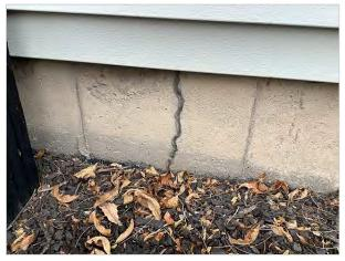
Sealed crack observed on front foundation wall - no water intrusion found on inside wall surface (crawl space)
