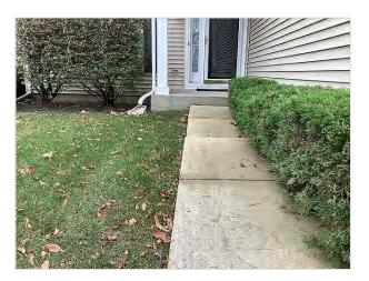
**Trip hazard present on the walkway to the front entrance**. The hazards can be repaired using a suitable or similar surfacing material to "feather" the out-of-level condition to make a smooth transition.
