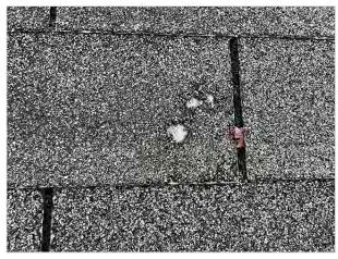
Aggregate worn through - fiberglass reinforcing fibers visible
