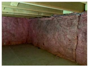
Crawlspace walls insulated with batted fiberglass
