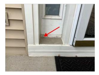
**Exterior caulking penetrations is cracked or missing.** The caulking should be repaired or replaced to help prevent water intrusion.
