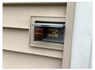
GFCI functions well however electrical outlet box is loose and needs to be resecured
