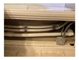
The GFCI for the jetted tub was not located. The buyer should consult with the seller to determine if such a circuit exists. If none is present, a dedicated GFCI should be added to the jetted tub prior to use. This is a potential safety
