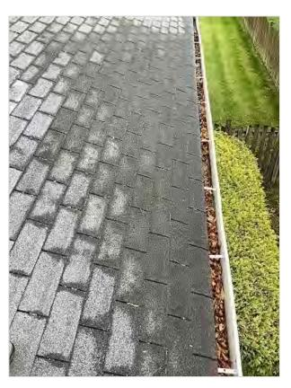
Some of the downspouts are missing and draining improperly onto the roof. HomeTeam recommends ensuring termination points for all downspouts are extended directly into the roof gutter system to prevent premature wearing of roofing materials and configured in such a manner to ensure all water flows away from the foundation during periods of rain.
