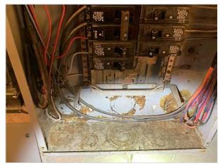
Corrosion at bottom of electrical panel
