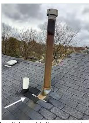
Newer shingles around plumbing and gas exhaust vents
