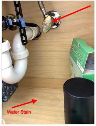
Upper level hall bath - left sink - cold water supply line shutoff valve leaks when turned on - currently turned off to prevent leaking
