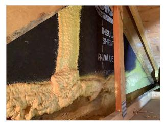
Spray foam insulation at seams between garage and main home
