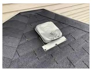
Roof vent above garage partially crushed
