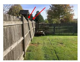
Main fence vertical supports weak and failing - fence loose and swaying away
