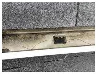
Missing downspout - gutter draining directly onto roof below
