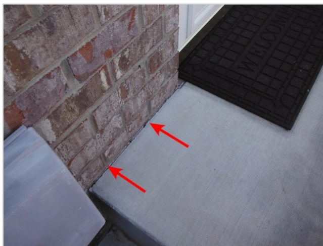
Open joints-Right
