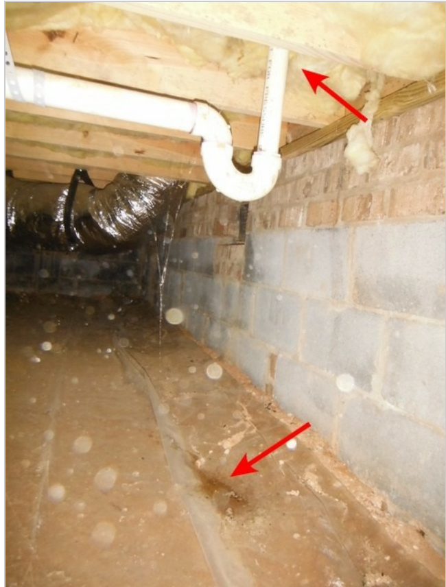
Leaking-Jetted tub
