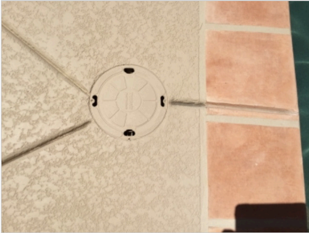
Cover Painted in Place
