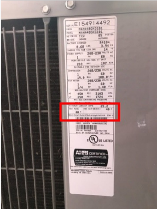
Outdoor Unit- Max Fuse 40 Amp
