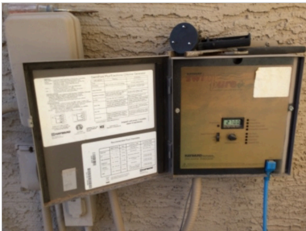
Salt Cell Control Box
