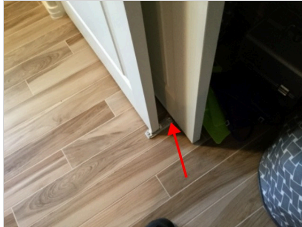
Left Front Bedroom Closet
