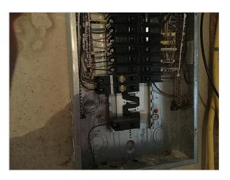
The visible house wiring consisted primarily of the Romex type and appeared to be in good condition. An electric service grounding system was installed. Service grounding requirements have changed many times over the years. The grounding system for a 30-year-old electric service is different from that of a 10-year-old service. The inspection does not attempt to verify that the grounding system or any other part of the electric service complies with current codes.
