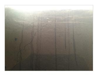
Cracks in the basement show signs of previous water intrusion. Below grade cracks are highly susceptible to water intrusion during times of heavy rain. The cracks should be monitored to determine if they are active. If a waterproof basement is required, HomeTeam recommends having the cracks sealed to prevent water intrusion.
