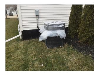
The cooling system was visually inspected but was not tested due to cold exterior temperatures. When outdoor temperatures have been below 60 degrees F within the preceding 24 hours, operation of the cooling system can damage the compressor. Full functionality will need to be evaluated when the outside temperature remains above 60 degrees. The system should be cleaned, serviced, and inspected by an HVAC technician in the spring.
