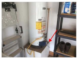
There was no sediment trap present on the gas line. You should consider having one installed to help prevent potential debris from entering the gas valve.
