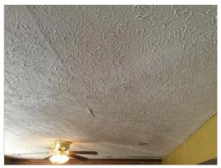
Past patching/repairs were visible at the garage ceiling at the rear left.
