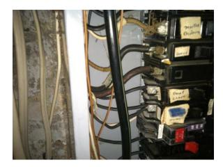
There were circuit breakers in the main electric panel that had two attached circuits. Each circuit should have its own dedicated breaker to prevent nuisance tripping and good terminal contact. One of the wires should be removed and connected to its own appropriately sized breaker by a licensed electrician.
