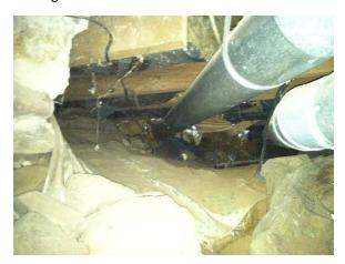
The surface of the ground was not entirely covered with a moisture barrier. A polyvinyl (minimum 6 mil) moisture barrier should completely cover the ground to keep the crawlspace dry. Crawlspace moisture can lead to wood rot and/or mold growth that could damage the floor property and pose health risks.
