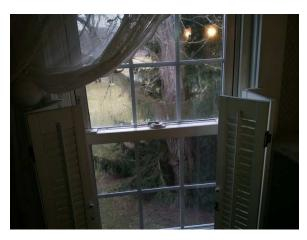
The seals on a representative number of windows (2-3+) in the home had failed causing a loss of vacuum between the panes and a resulting loss of insulation value. The most noticeable result of this failure is condensation and fogging between the panes of glass.
