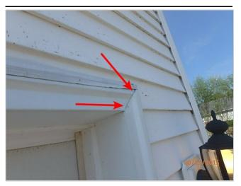
Garage door's aluminum wrap installed improperly
