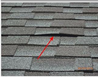
Nail pops lifting shingles on front roof
