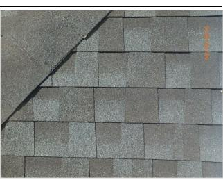
The roof requires routine maintenance to prolong its life (nail pops on front of roof).
