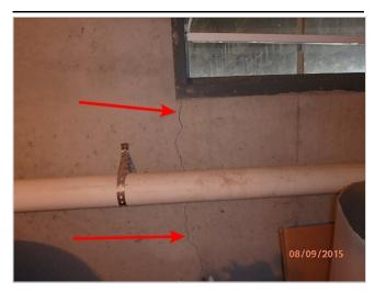
View of foundation crack from basement window
