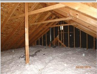
Parts of the attic show signs of previous water intrusion. The areas were dry at the time of the inspection. The buyer should maintain vigilance in monitoring the areas for any recurrence of the previous issue and should rectify any issues immediately upon observing them.
