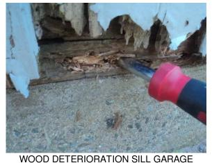
• We observed significant wood deterioration of the windows on the left side and in the rear of the garage.
