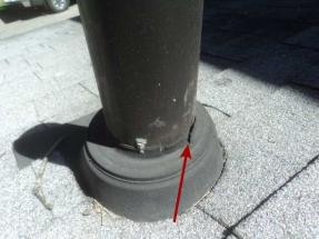
CRACK IN PLUMBING VENT FLASHING
