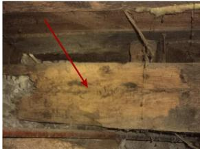
DETERIORATED BEAM IN CRAWL SPACE
