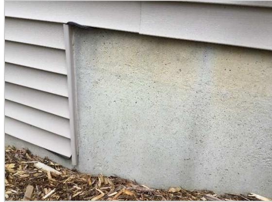
Small cracks were observed on the foundation. The cracks were 1/16th-inch or less in width. The homeowner should monitor these cracks for any changes, and if changes are noted, should contact a structural repair company for further analysis. Below-grade cracks are highly susceptible to water intrusion during times of heavy rain. Water staining from previous water intrusion was not visible. HomeTeam recommends sealing these cracks if a watertight basement is desired.
