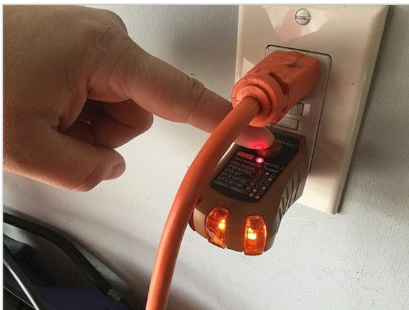
**One receptacles in the garage have hot and neutral wires reversed.** This is a safety concern and should be repaired and further assessed by a licensed electrician. Please note that we only test outlets that are visible and readily accessible at the time of the inspection.
