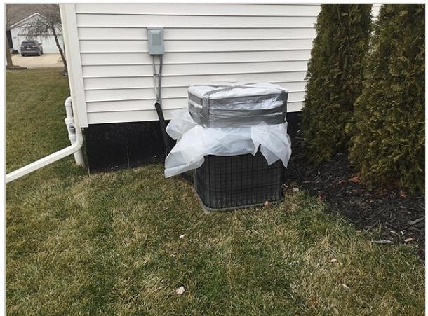
The cooling system was visually inspected but was not tested due to cold exterior temperatures. When outdoor temperatures have been below 60 degrees F within the preceding 24 hours, operation of the cooling system can damage the compressor. Full functionality will need to be evaluated when the outside temperature remains above 60 degrees. The system should be cleaned, serviced, and inspected by an HVAC technician in the spring.
