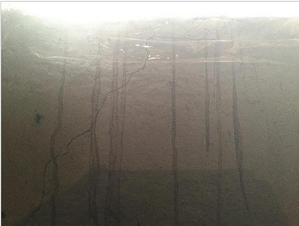
Cracks in the basement show signs of previous water intrusion. Below grade cracks are highly susceptible to water intrusion during times of heavy rain. The cracks should be monitored to determine if they are active. If a waterproof basement is required, HomeTeam recommends having the cracks sealed to prevent water intrusion.
