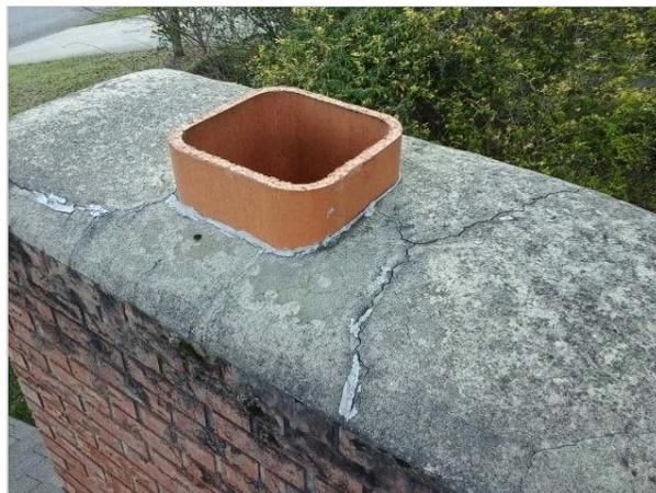
*There was typical sealant/patching visible around the chimney/flashing area. Any areas where patching has occurred is an indication of past/active leaks and should be monitored periodically for drying out or cracking of the sealant used.*
