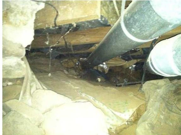
The surface of the ground was not entirely covered with a moisture barrier. A polyvinyl (minimum 6 mil) moisture barrier should completely cover the ground to keep the crawlspace dry. Crawlspace moisture can lead to wood rot and/or mold growth that could damage the floor property and pose health risks.
