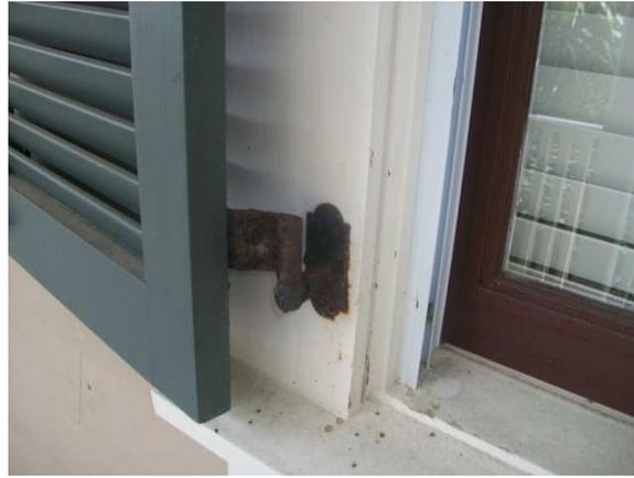
A representative number of the windows were painted shut and could not be operated to verify operation or check for defects. The window(s) need maintenance to free them for opening and further inspection.
