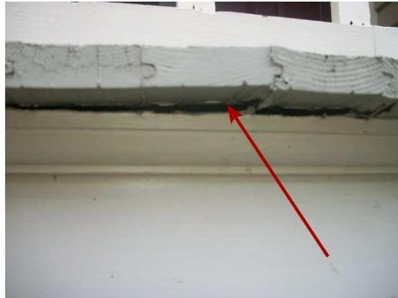
Some areas of right side porch 1st floor has moisture damage to railing/lattice work. Consult Contractor for further evaluation.
