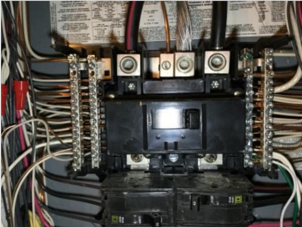
**Evidence of amateur wiring was observed in the garage.** Amateur wiring may not conform to standards methods and could be a safety concern. Consult with a qualified electrician for repairs and further evaluation.
