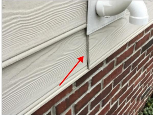
**Rotted or weather damaged wood was present on many areas of the exterior of the home.** The areas should be repaired and further evaluated at the time of repair.
