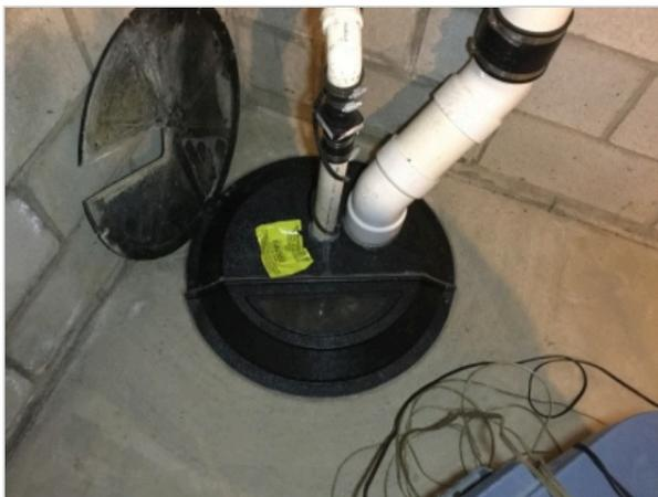
Exterior sump pump discharge line has a gap. Recommend to repair as necessary.
