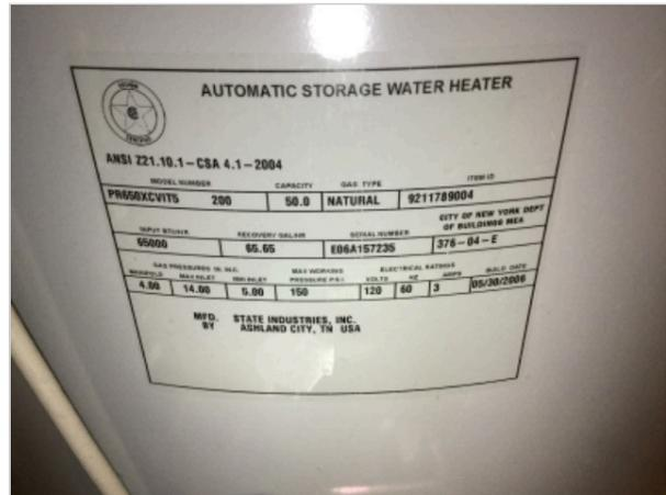
The water heater may be past its design life. This is an informational note only to help give an idea of future budgeting considerations. The unit was functional unless noted otherwise. Please note that since codes change, it is possible the configuration for a water heater's flue and/or discharge may need to be altered at the time of a future replacement.
