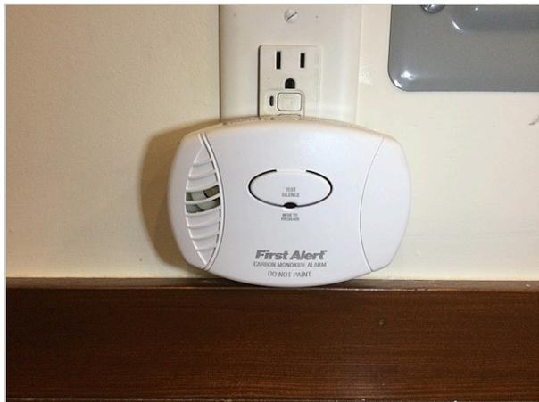
Per Colorado state law, carbon monoxide detectors are required to be installed within 15 feet of all sleeping areas. No carbon monoxide detectors were observed installed within 15 feet of the sleeping areas on the upper level.
