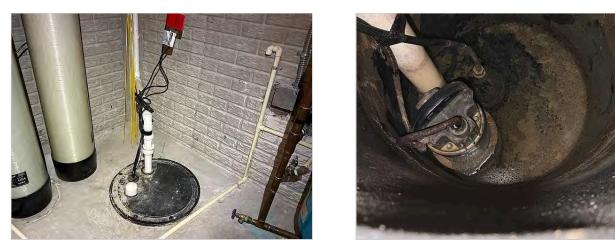
An ejector or grinder pump is installed in the home. The purpose of the ejector pump is to eject raw sewage to the main sewage line located at a point higher than the location of the pump. These systems are found in the lower level of homes situated below the main sewer line. Ejector pumps are sealed with a majority of their plumbing systems not visible for inspection. HomeTeam recommends consulting with a qualified plumbing contractor for more information as needed.
