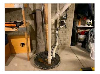
The pump cover for the ejector pump in the basement is rusted. This condition can allow for gasses from the wastewater in the crock to enter the living area of the home. For proper functionality, HomeTeam recommends the pump cover be resealed.
