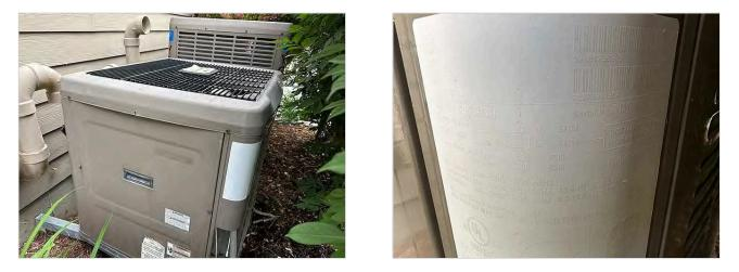
The second electric outdoor air conditioner condensing unit was a York, Model Number CZF04813CA and Serial Number W1C1859086. The unit is located on the left side of the structure. This unit is approximately 12 years old. Periodic preventive maintenance is recommended to keep this unit in good working condition. The air conditioning system was tested and found to be functional but in need of service.
