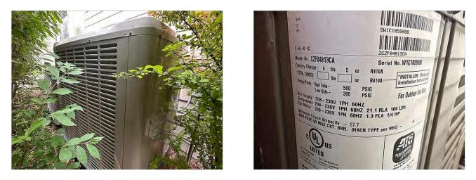
**The temperature differential for the air conditioning units was approximately 9 to 14 degrees which is inadequate.** Typically an air conditioning unit should have a temperature differential of approximately 16-22 degrees. To help improve the efficiency and performance, HomeTeam recommends consulting with a qualified HVAC technician for further evaluation and options on repair, recharge, or replacement.
