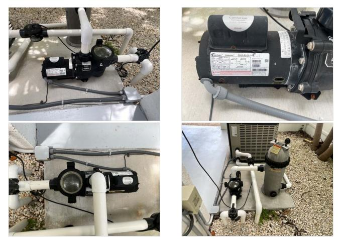
The Jandy pool cartridge filter was operational at the time of the inspection. The efficiency of the filtration system is not within the scope of the inspection. All pool filters require cleaning and routine maintenance in order to properly clean the water. Consult with the manufacturers documentation for maintenance procedures.
