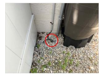
There was corrosion on the electrical service entrance box. Maintenance would be recommended in order to access the main breaker with ease whenever needed.
