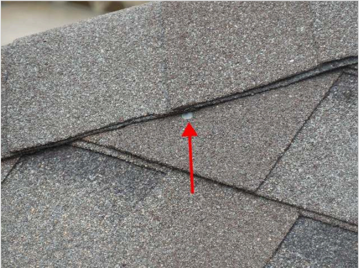
Exposed nail head on roof.
