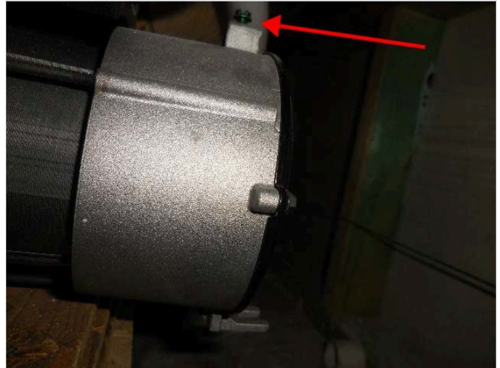
Spa tub motor not bonded.
