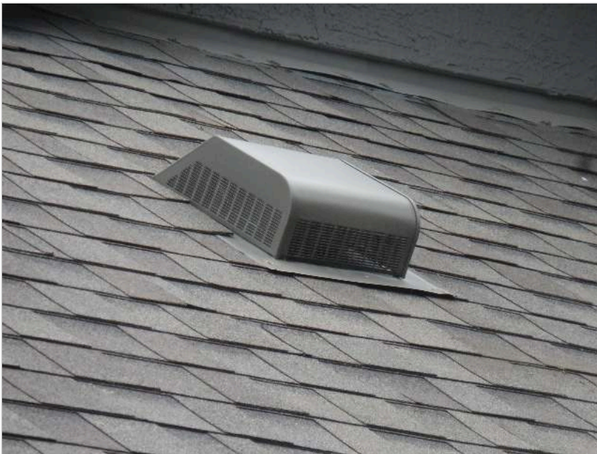
Screened dryer vent cover.
