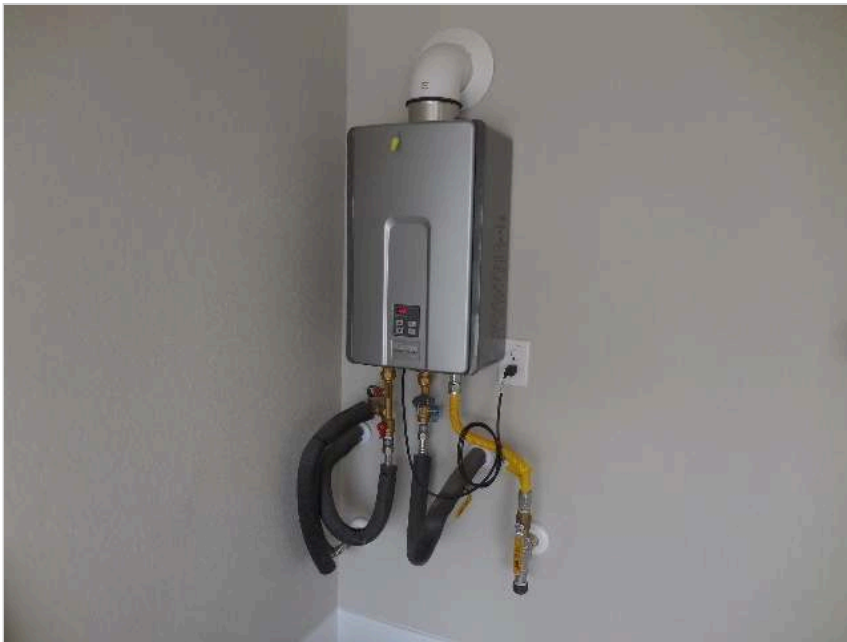
View of tankless water heater in garage.
