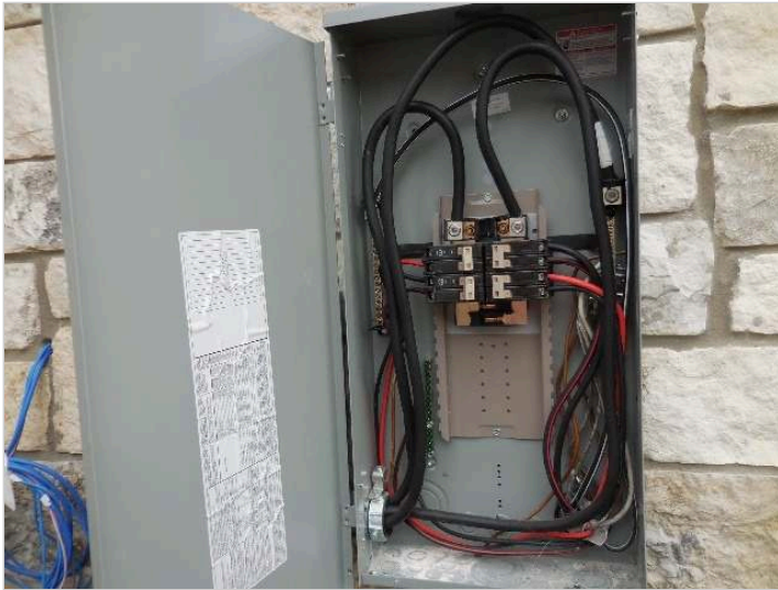
View of main electrical panel.
