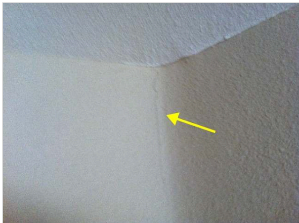
Minor settlement cracks
