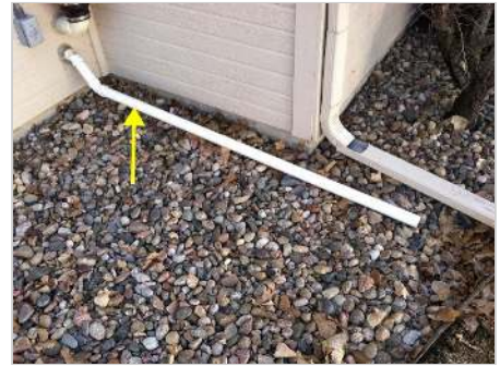
Sump pump discharge pipe
