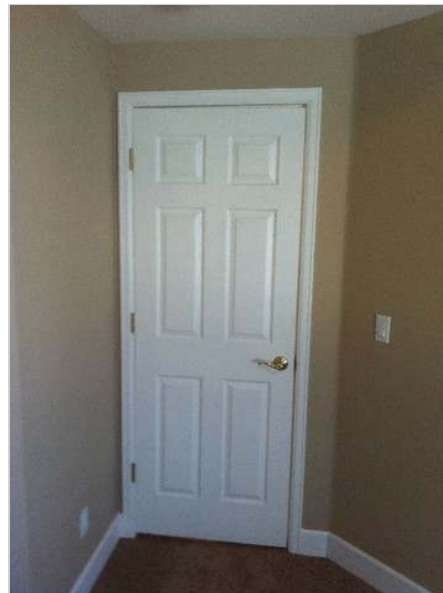
Basement bedroom door somewhat out of alignment. The door was functional during the inspection.
