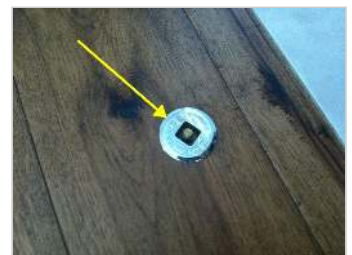
Gas shutoff valve for fireplace
