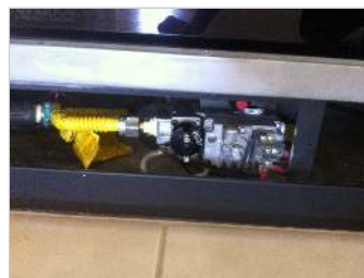
Controls for gas-log fireplace
