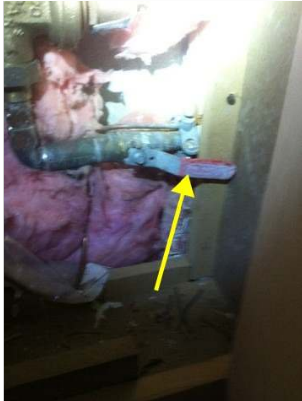
Main water shutoff valve
