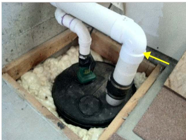
Radon mitigation pipe installed in basement sump
