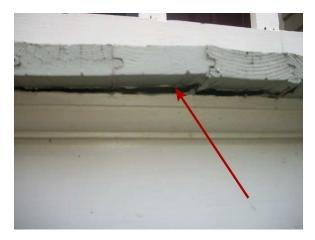
Some areas of right side porch 1st floor has moisture damage to railing/lattice work. Consult Contractor for further evaluation.
