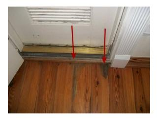
Moisture damage under windows on interior walls in dining area and 2nd floor rear den window(s)
