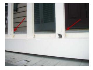
Moisture damage front and side porch 1st floor to trim along bottom under decking
