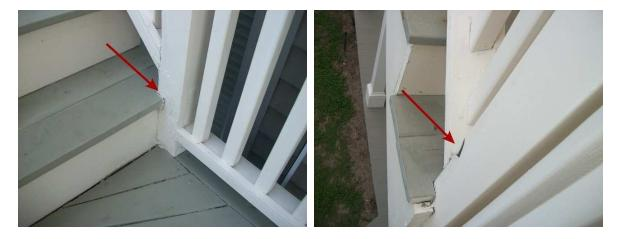
Wood to ground moisture damage visible on right side of home. Consult Contractor for further evaluation
