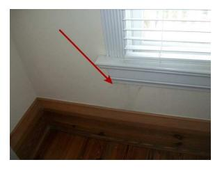
Moisture damage right side 2nd floor entry door/casing/trim
