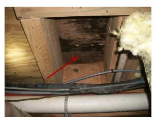
There are several areas of plywood /insulation under home covering floor structure missing. Areas should be repaired to prevent rodent entry into floor structure.
