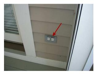
Pool electrical light switch mounted on face of rear porch loose and needs to be re-secured
