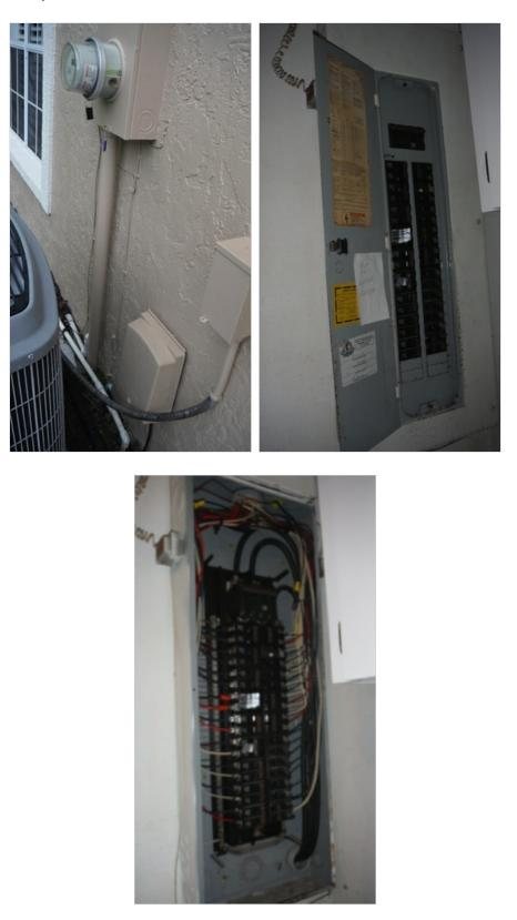
The electric panel is surrounded by cabinets and is not immediately accessible. This could create an unsafe condition in the event of an emergency.
