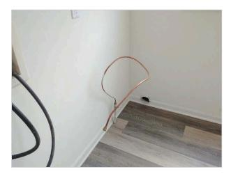
The refrigerator water line was not capped. Water lines need to be capped after a shut off valve or leaks could occur.
