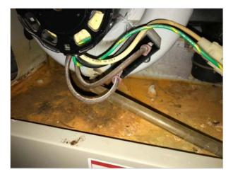
When the burners fired up there was roll out (flames). The burners may be plugged. The safety switch in the blower housing sticks. Further evaluation is recommended prior to closing.
