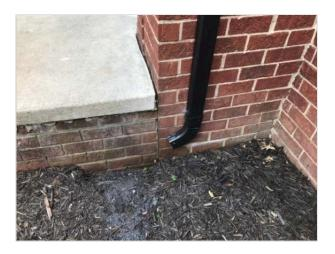
The gutters need to be cleaned. Clogged gutters can cause roof drainage water to back up and cause damage to the structure, soffit and fascia. Keeping gutters clean will help move water away from the foundation which could lead to basement water problems.
