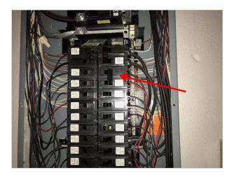
The visible house wiring consisted primarily of the romex type and appeared to be in good condition. An electric service grounding system was present.
