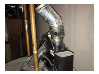
The T&P valve on the water heater was leaking at the time of the inspection. If the water pressure and temperature within the unit are within the normal range the valve may defective.
