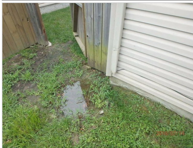
several downspouts are draining adjacent to the foundation
