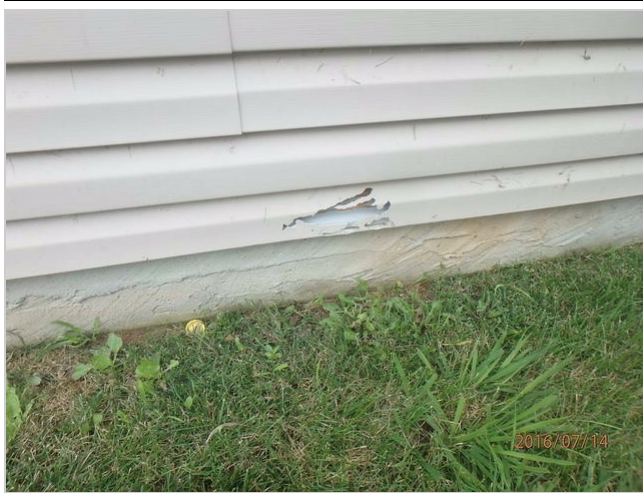
example of damaged siding
