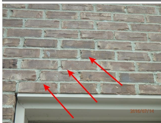
mortar crack
