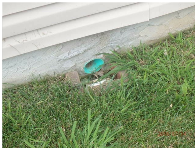
missing dryer vent cover
