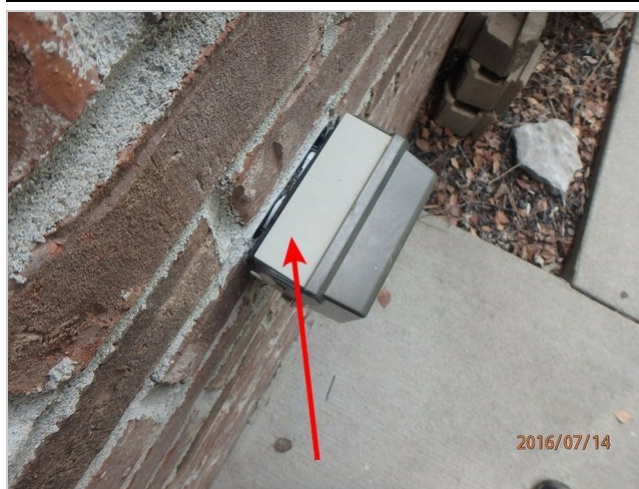
outlet is not properly covered
