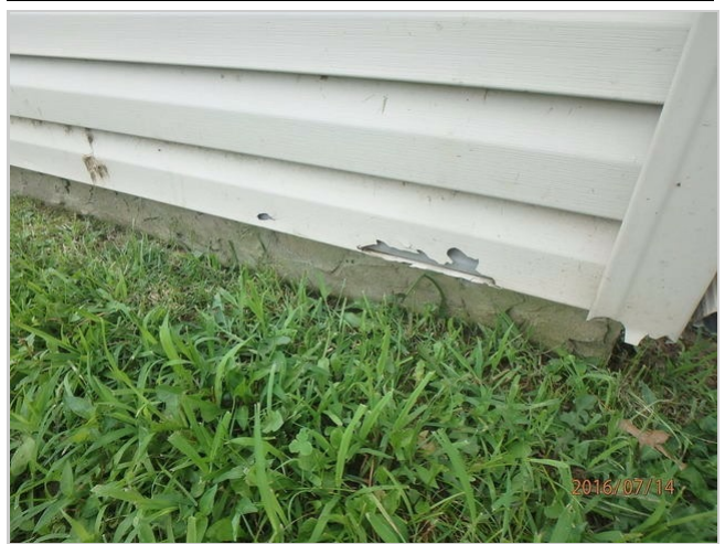
example of damaged siding
