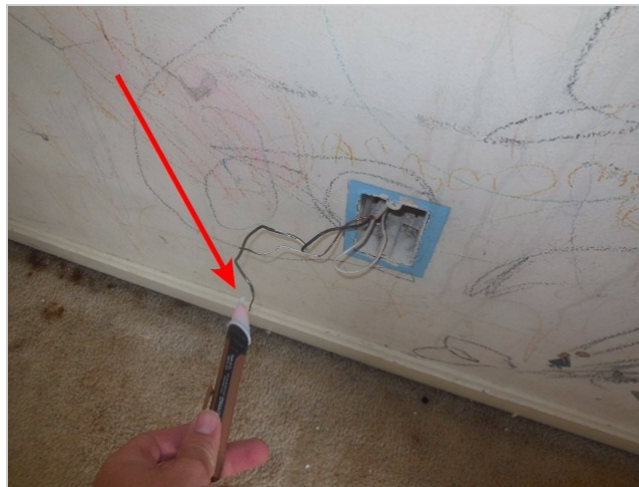
Exposed live wires.
