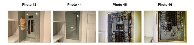
**Circuit breakers in the electric panel had two attached circuits (wires)**. Each circuit should have its own dedicated breaker to prevent nuisance tripping and ensure good terminal contact, which may help prevent overheating. This situation is commonly referred to as a "double-tap". Recommend that an electrician repair this condition and further assess the panel for any additional required repairs.
