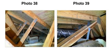
**Cut truss(es) observed in the attic.** This is a support/installation/damage concern. Typically, truss modifications/ repairs are to be approved by the manufacturer or structural engineer. Modifications to trusses can alter the design load. Recommend review and repairs as directed by a structural engineer with repairs performed by a qualified contractor.
