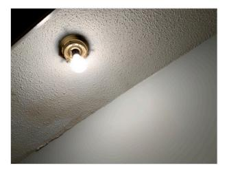
The overhead ceiling fan/light in the front bedroom were not operated by a light switch.
