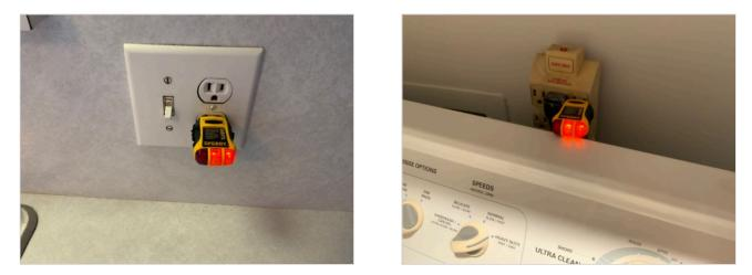
A blocked opening was observed in the electrical outlet in the living room. This is a damage/safety concern. Recommend repair by a qualified person.
