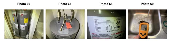
The hot water temperature was greater than 125F and may pose a risk of burning. HomeTeam recommends adjusting the hot water temperature by turning down the water heater thermostat.
