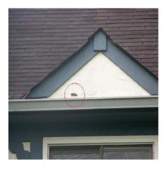
NOTE: The top left dormer has areas of stucco that need to be sealed. The rear right side of the home, where the stucco meets the cedar one by six wood trim, needs to be sealed. The rear door frame for the sliding door has areas that need to be monitored and/or sealed.
