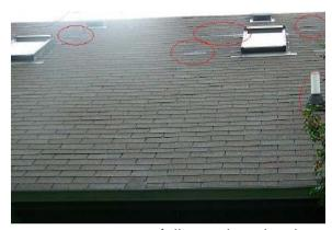
There were a represented of shingle tabs missing throughout the roof at the time of the inspection. Missing shingle tabs is not necessarily a sign of a roof leak. Consult with a qualified roofer to make repairs.
