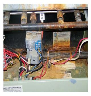
The home was heated by Rheem natural gas forced air furnace. The unit was located in the basement of the home and has an approximate input heating capacity of 100,000 BTUH.
