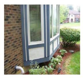
NOTE: The rear bay window should be sealed where frame meets brick siding.
