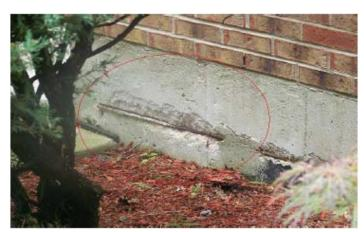
NOTE: The right side of home has an area on the concrete foundation that should be sealed.
