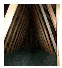
The attic was accessed through a scuttle in the 2nd floor bedroom closet. The attic above the living space was insulated with blown insulation, approximately 6-inches in depth.
