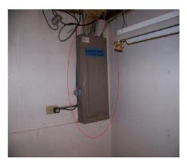
NOTE: Cover plate for the service panel box needs to be properly secured to the panel. There is a double tapped breaker in the service panel box. The basement ceiling has a receptacle that should be properly installed into a junction box.
