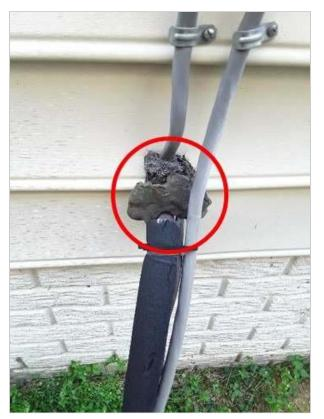
The insulation on the exterior air conditioning line set is dry-rotted. This could affect the efficiency of the system and should be replaced.
