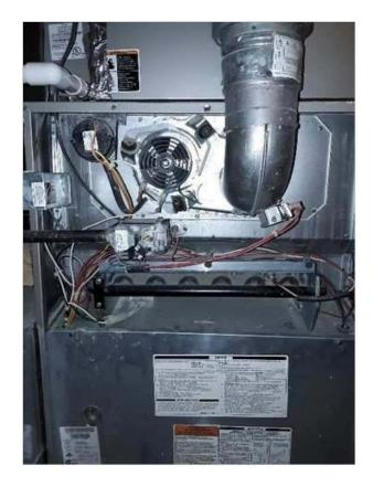
The average gas furnace will last about 15 years before needing to be replaced. A gas furnace will last longer by doing regular maintenance. The subject gas furnace has been in service for approximately 13 years and may be at or nearing the end of it's usable life.
