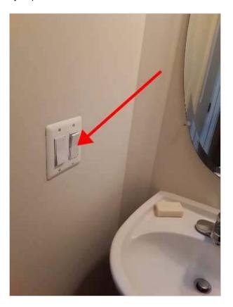
One or more devices were missing a switch/junction box/outlet cover in the mechanical/plumbing room. All switch/outlet boxes should be properly covered to avoid a shock hazard. Electrical related repairs should be performed by a qualified electrician.
