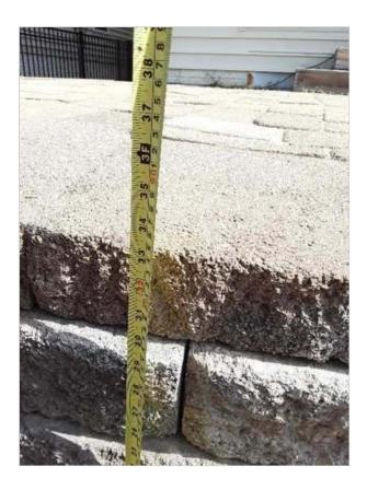
There were no handrails on the steps leading to the patio. This can pose as a safety concern for falling.
