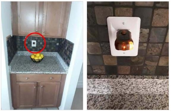
2. A broken switch was noted in the main level half bath. This could be a shock hazard due to exposed electrical contacts. The affected outlet(s) should be replaced by a qualified contractor.
