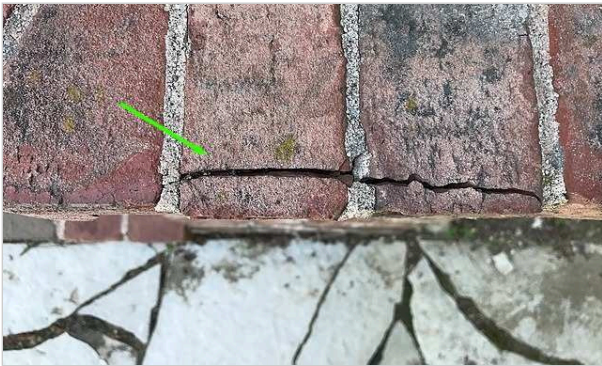
cracked bricks / mortar near the front door
