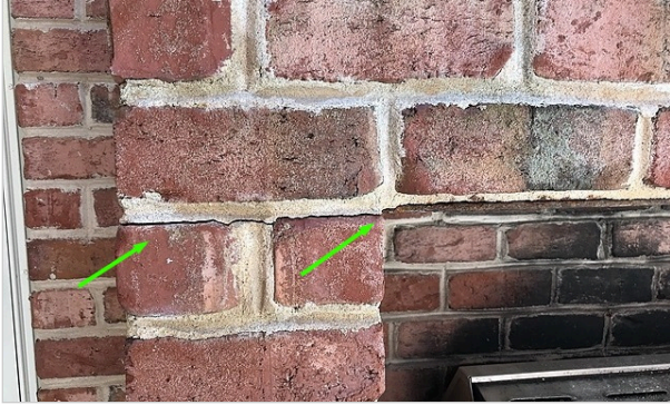
cracked mortar at the lintel line on rear grill chimney
