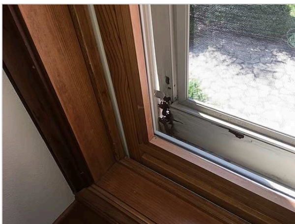
Wood rot in rear window.
