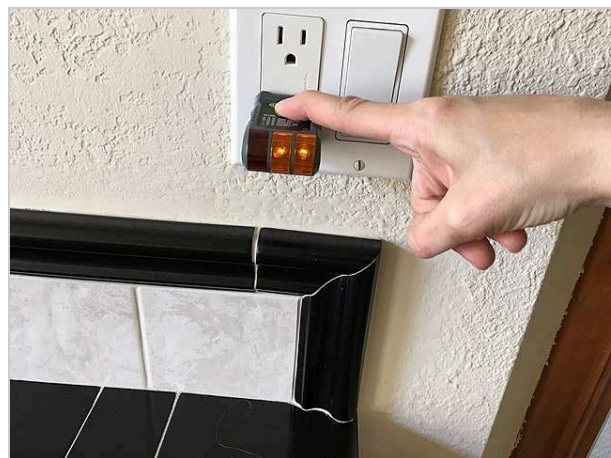
Master bath outlet right side not gfci.
