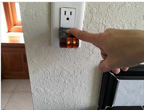
Master bath outlet left side not gfci
