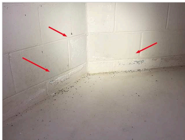
efflorescence - prior water noted right side basement
