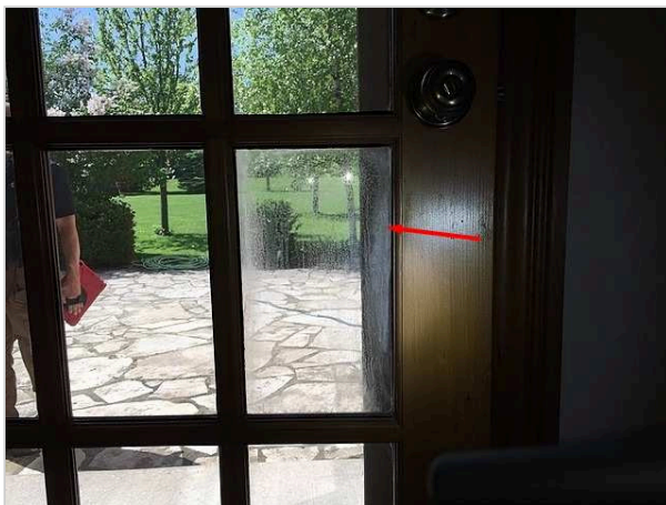
bad seal on rear patio door window pane
