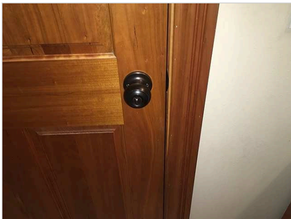
Hall bath door to the right upstairs does not latch.
