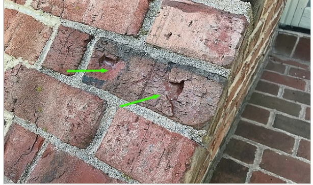
spalling of the brick near front entrance
