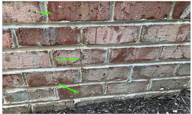
small cracks front right off walkway
