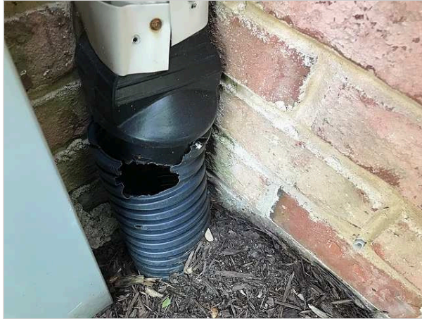
Torn downspout extension allowing water to drain too close to foundation
