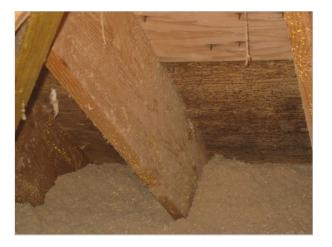
• One of the support columns on the far left side of the attic space was completely loose and needs to be secured.
