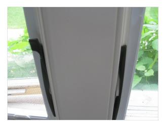
• The attached garage front window edges were bare wood that should be treated to prevent eventual wood rot.
