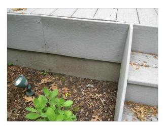
• There was movement and gaps along the outside trim boards for the deck that should be monitored for action.
