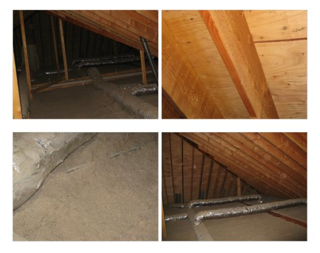
• There was darkened sheathing, with possible light mold growth, in the right front section of the attic that should be further evaluated and treated as necessary.
