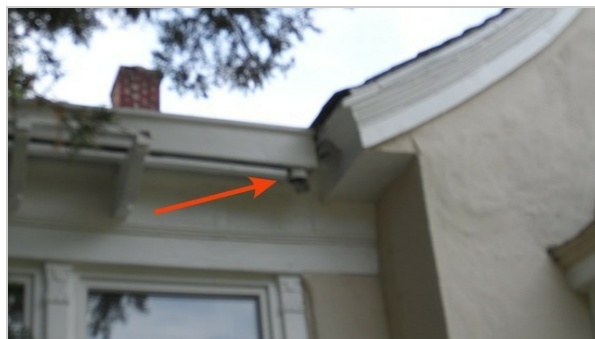
Missing downspout
