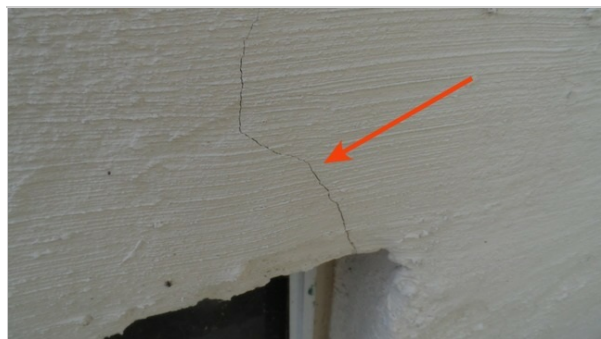
Minor cracking of stucco
