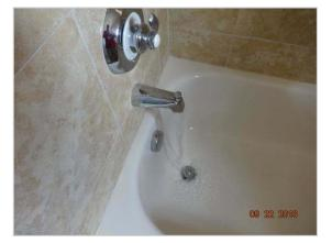
Plumbing fixtures should be adequately sealed/caulked at all wall and cabinet joins to prevent moisture penetration which could lead to the premature deterioration of adjacent surfaces and framing components, and may contribute to conditions conducive to the promotion of mold growth.
