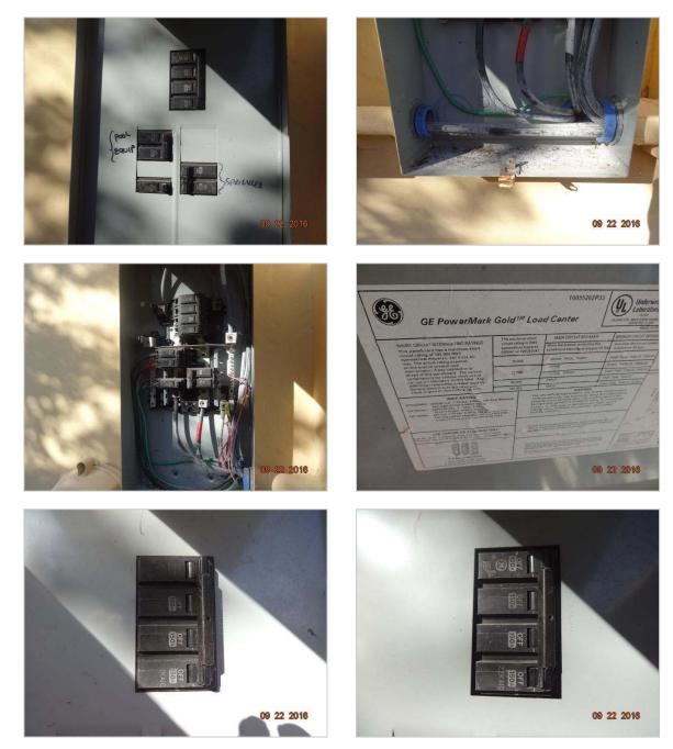
There was a legend inside the panel. The accuracy of the labeling was not determined. Accurate labeling allows individuals unfamiliar with the equipment to operate it.
