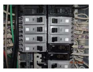
The visible wiring consisted primarily of Romex and did appear to be in serviceable condition.
