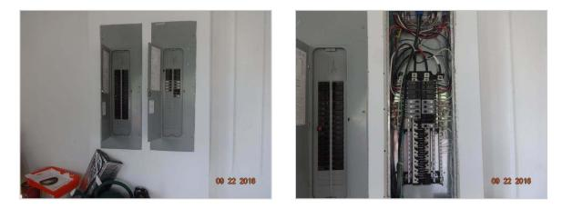
There was a legend inside the panel. The accuracy of the labeling was not determined. Accurate labeling allows individuals unfamiliar with the equipment to operate it.
