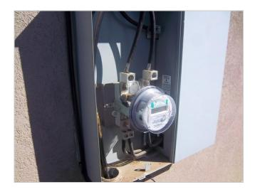
The weather tight main disconnect sub-feeds a Square D Homeline breaker type sub-panel located on the garage wall and an identical 200 amp breaker panel located in the basement and rated at 200 amps of capacity each.
