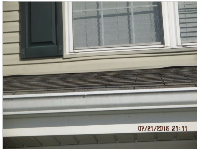
Loose flashing
