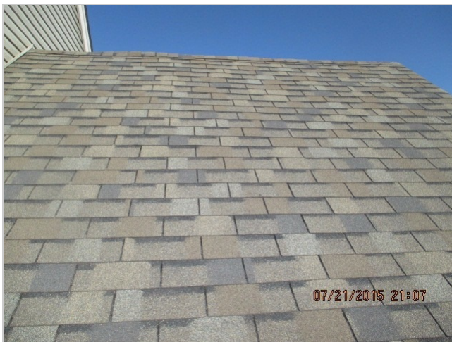
Right side roof
