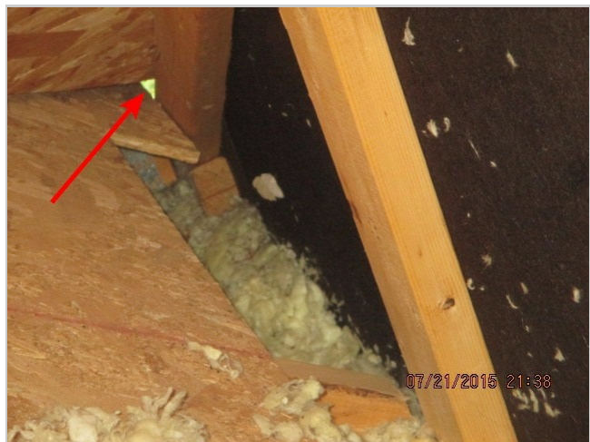
Opening from attic side
