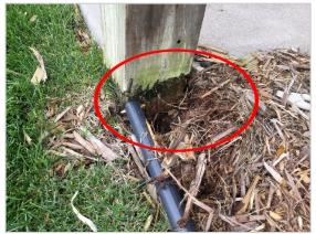
Monitor deterioration of deck support and repair/replace as necessary.
