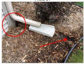
Back left downspout has a hole where water was running near house and mulch is washed out from today's rain.
