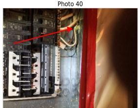
Corrosion present on wires. Appears dry at this time.
