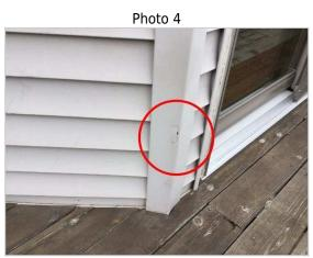
Damage to siding on back deck.
