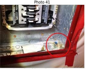
Corrosion drips at bottom of box.
