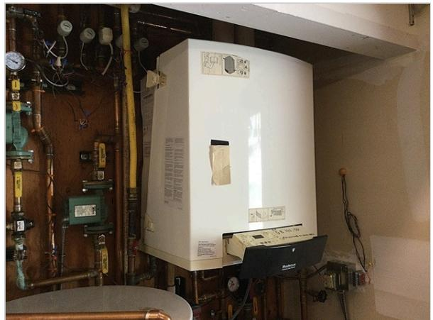
Corrosion was observed on the water distribution pipes for the hydronic heating system. No water leaks were observed at the time of the inspection.
