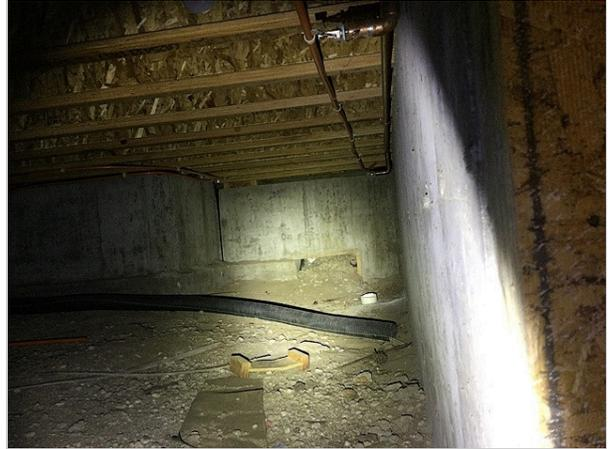
**The sub-floor above the crawlspace lacks insulation.** Adding insulation may help regulate the temperature of the living space above the crawlspace and may assist in preventing moisture intrusion.
