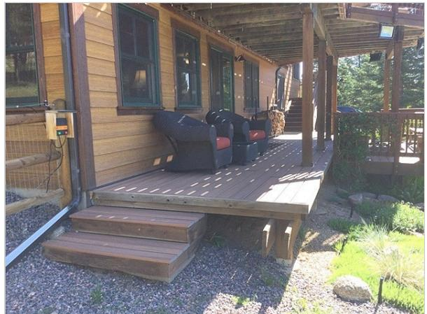
**The grading around the structure appears to be insufficient to carry water away from the foundation.**
