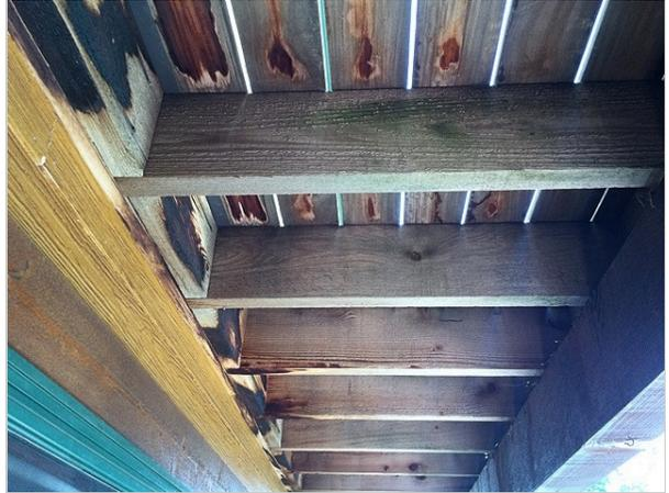
A few of the joist hangers on the middle deck appear to be coming loose. Recommend repairs by a qualified contractor.
