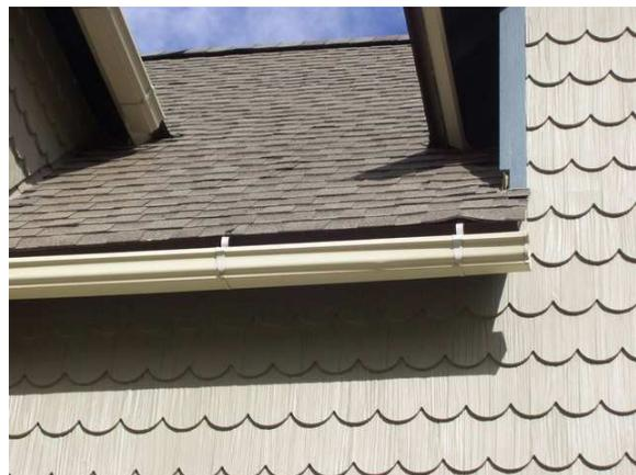
There was light curling and moderate surface wear observed on the roof shingles at the time of the inspection. These conditions indicate the roof shingles were in the middle stages of their useful life. This visual roof inspection is not intended as a warranty or an estimate on the remaining life of the roof. Any roof metal should be kept well painted with a paint specially formulated for the use. There were no major visual defects detected on the exterior of the roof.
