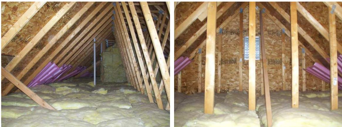
Because of the configuration of the framing and absence of a catwalk, which limited access, it was not possible to inspect all areas of the attic. There was no moisture visible in the attic space. The absence of visible indications of moisture is not necessarily conclusive evidence that the roof is free from leaks. The only way to be sure a roof does not leak is to inspect the underside of the roof during a heavy rain. There were no major visual defects observed in the attic or roof structure.
